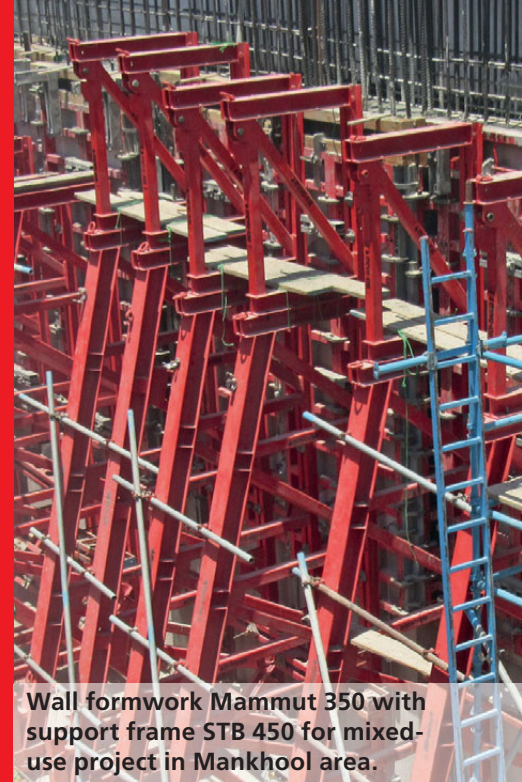
Wall formwork Mammut 350 with support frame STB 300 for mixed-use project in Mankhool area.
