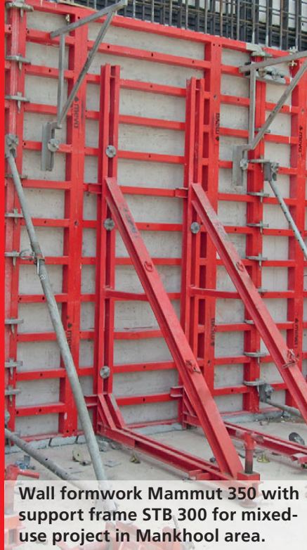
Wall formwork Mammut 350 with support frame STB 450 for mixed-use project in Mankhool area.
